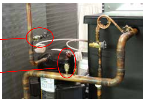
Typical placement of non-adjustable "fixed" pressure switches.
