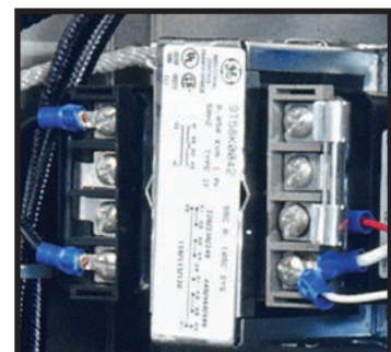
Typical control circuit transformer fuse
