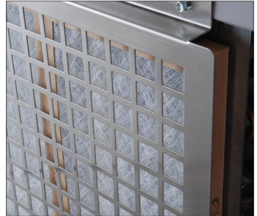
Detail of MERV 3 filter enclosed within a condenser screen.
