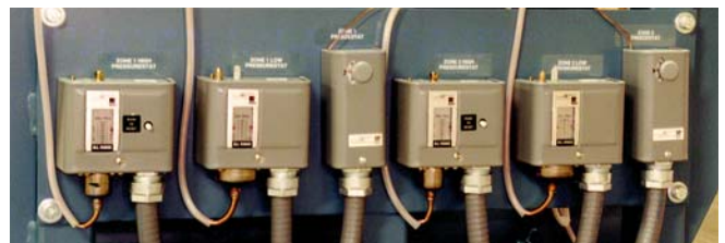
Typical use of refrigerant limit switches on Advantage central chillers.
