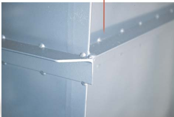
Close up detail of tank banding.
