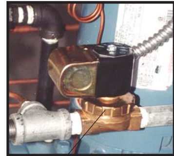
Make-up solenoid valve
