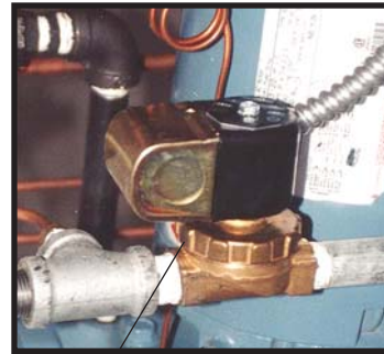
Typical water make-up solenoid valve Figure 5.4A
