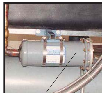
Typical filter-drier Figure 6.2C
