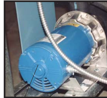
Pump Motor Assembly Figure 6.1A
