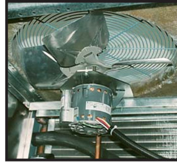
Typical fan assembly Figure 2.4A
