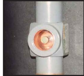
Refrigerant sight glass Figure 6.2D
