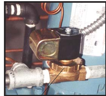
Make-up solenoid valve
