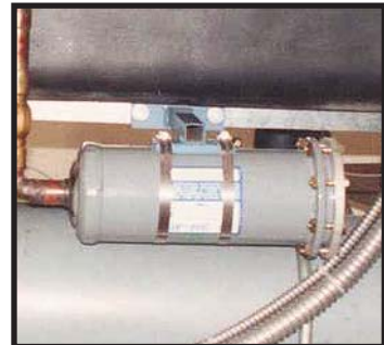
Typical filter-drier Figure 6.2D
