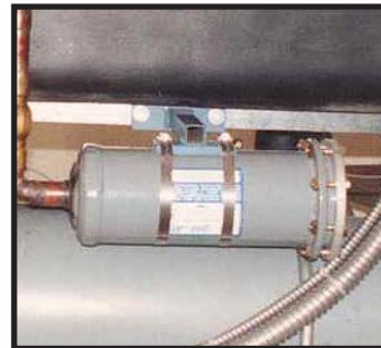
Typical filter-drier
