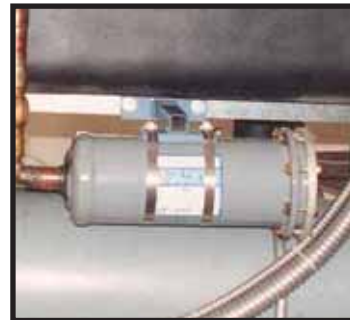
Typical filter-drier
