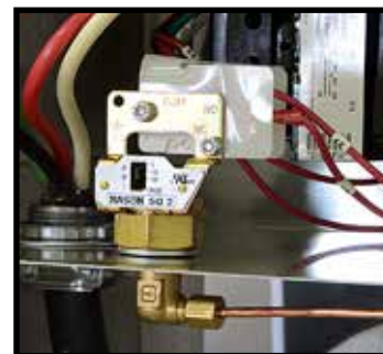
Panel mounted pressure switch
