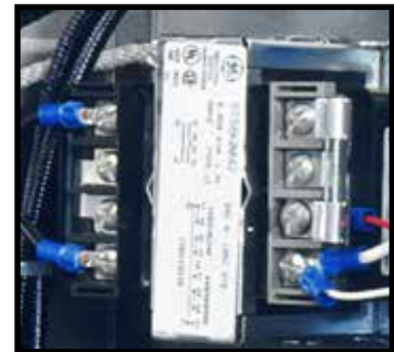
Control circuit transformer fuse
